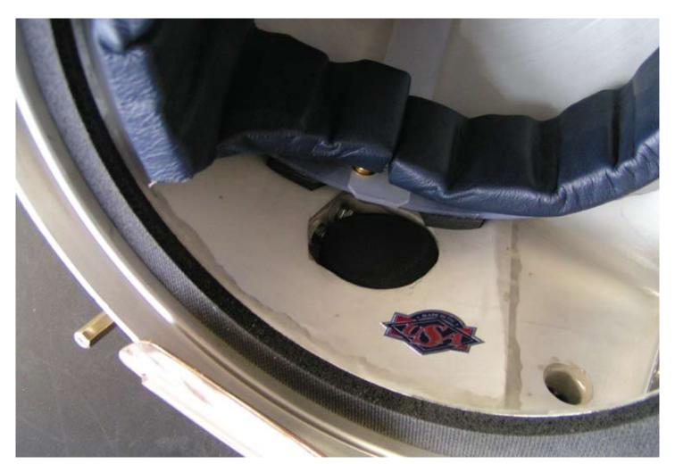
swool in the air diffuser for cleanliness and replace if necessary.
